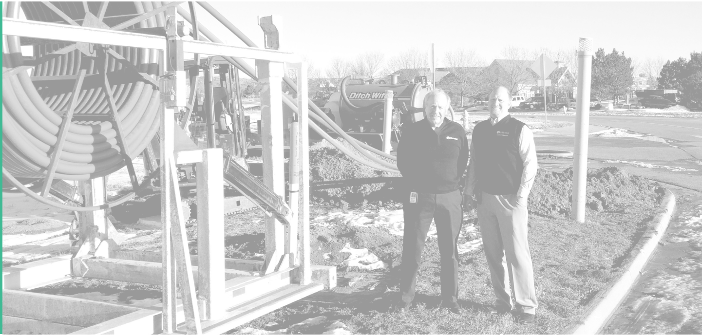
Construction of fiber backbone in Centennial, CO.
